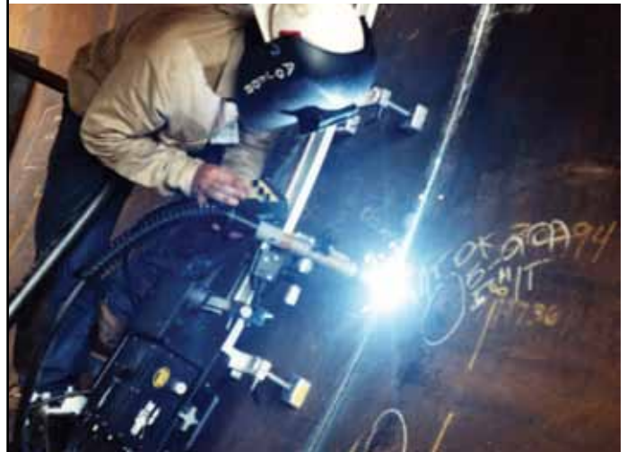
Shown Above - Vertical linear weave welding with ARM-2480 Support Bar w/ Magnets
